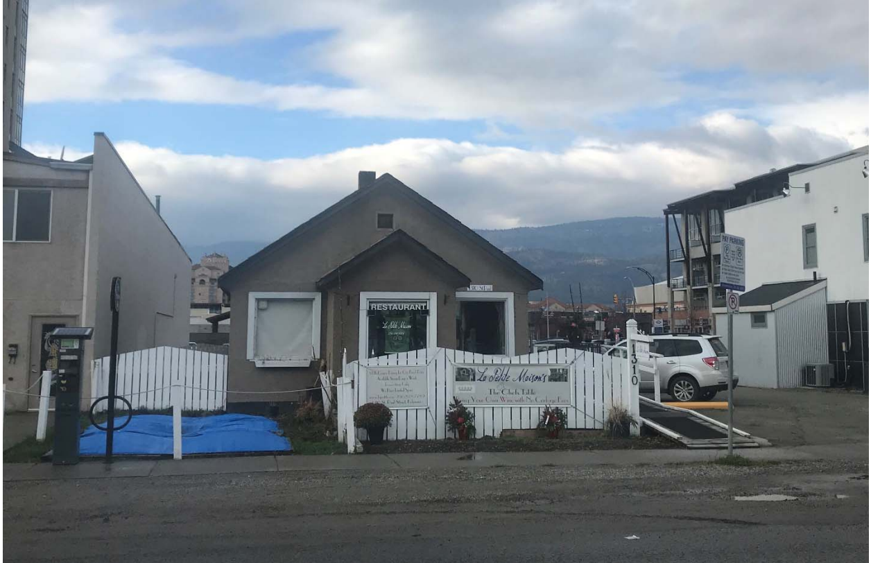
Looking west at front of existing building
